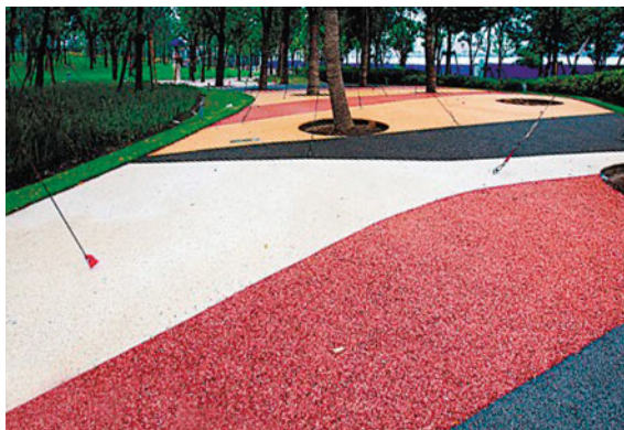
Fig. 2.129 Permeable pavement in the Expo site
