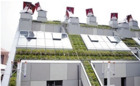
Fig. 3.20 Roof of London Case Pavilion
