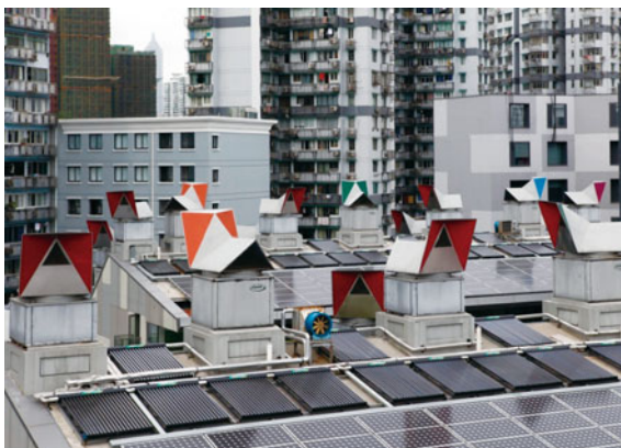
Fig. 2.83 Roof air caps in London Case Pavilion
