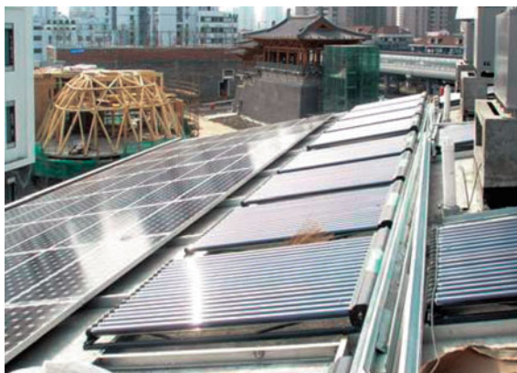
Fig. 2.9 Solar photo-thermal devices on the roof of Shanghai's UBPA case
