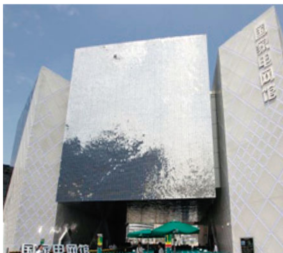
Fig. 2.99 State Grid Pavilion in the Expo
