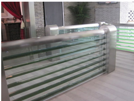
Fig. 3.21 Microalgae railing of Shanghai Eco-Home
