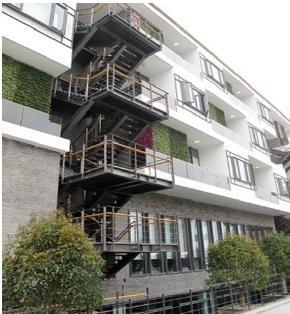
Fig. 3.23 Side wall greening of the Shanghai Eco-Home
