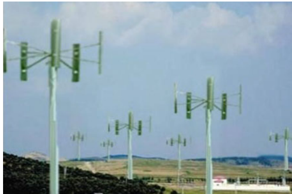
Fig. 2.23 Vertical axis wind turbine (VAWT)
