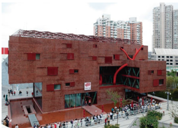
Fig. 2.61 Hamburg house in the Expo
