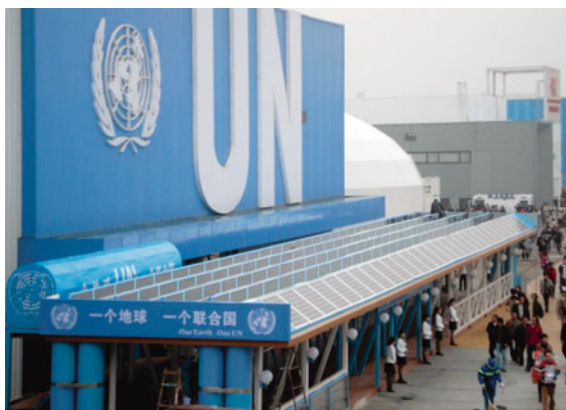
Fig. 2.10 Integrated solar thermoelectric system on the top of the waiting area of the UN Pavilion
