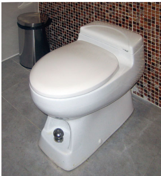
Fig. 2.123 The cup cleaner water-saving toilet in United Nations Pavilion
